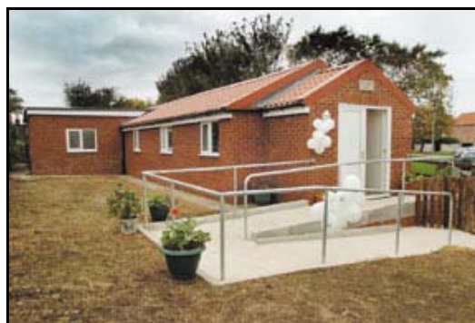
The newly refurbished WI Hall in Flamborough, East Riding
