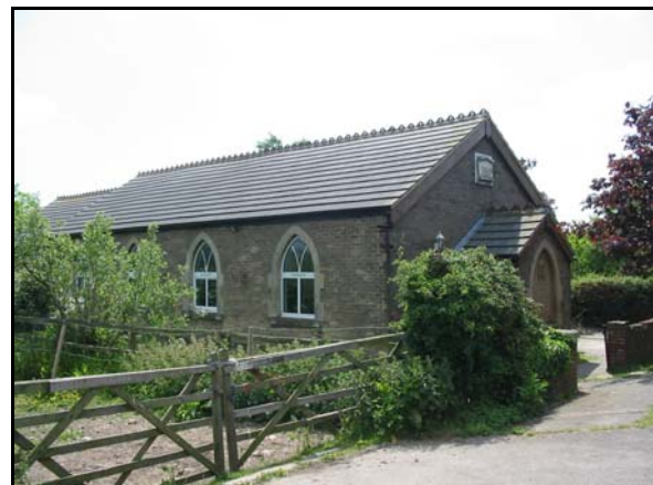
Habrough Village Hall North East Lincolnshire
